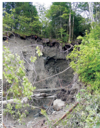
Bank erosion along Saint John River
